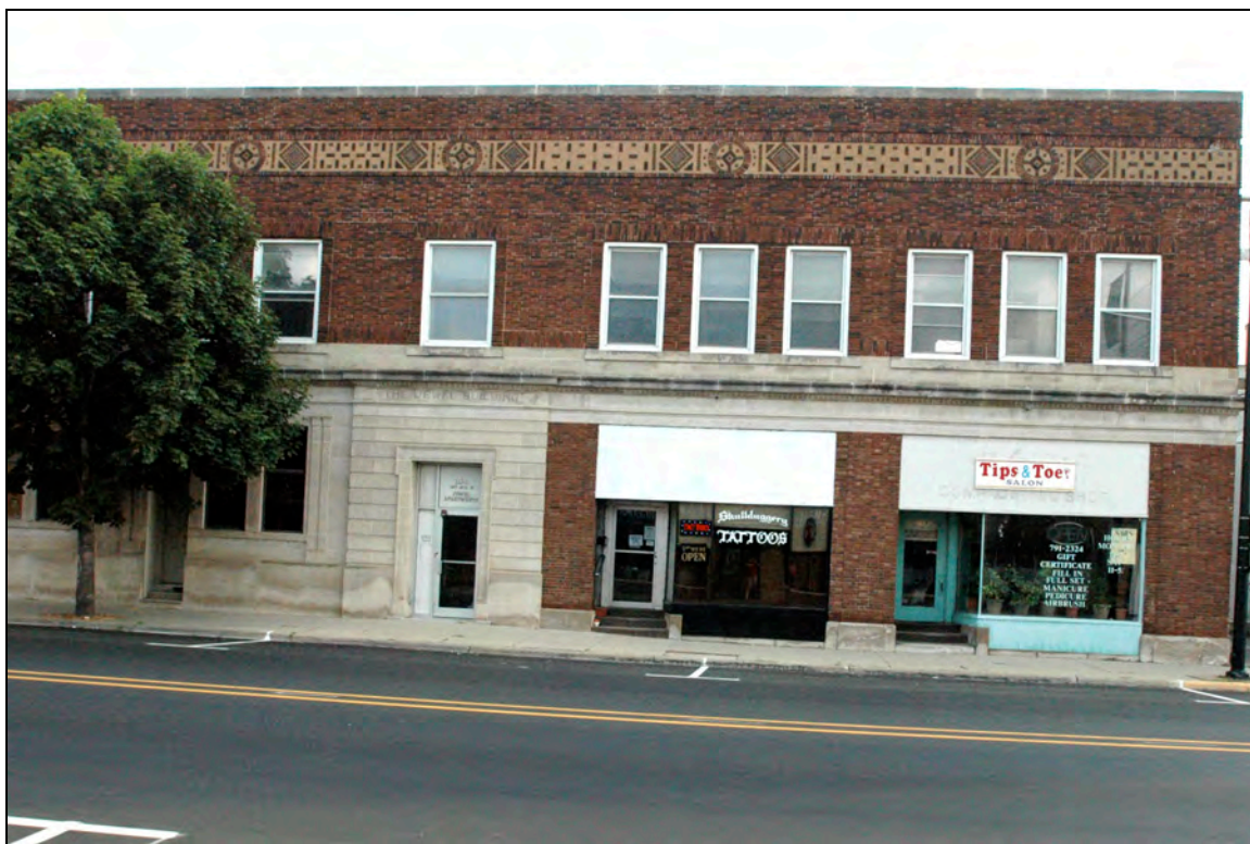
View of the south elevation of the Jewel Building looking north across 1 st Ave. E. The entrance to the upstairs apartments is numbered 104, and the two bays (from left to right) carry the numbers 108 and 110 1 st Ave. E.
