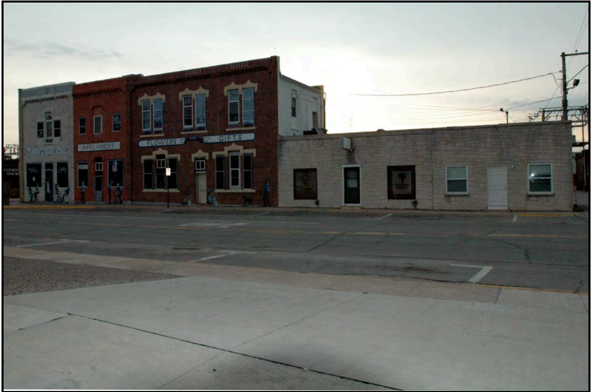
View of the west elevation, looking northeast across S. 3 rd Street showing the one-story addition.
