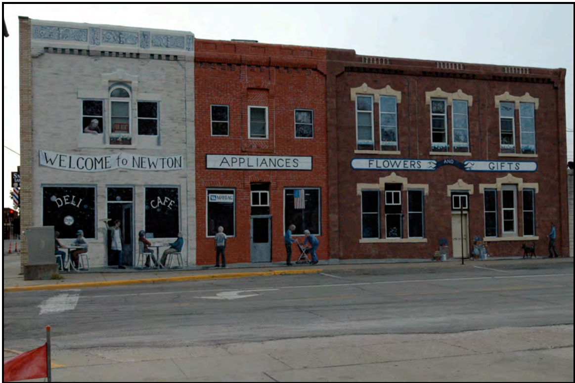
View of the west elevation of the original, ca.1885 building with the contemporary mural.
